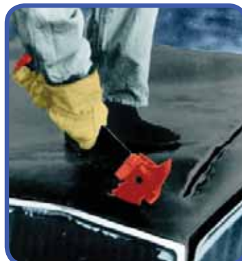
5. Leave some material in the corners until last.
