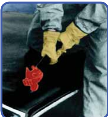
4. Chop close to the roof edge - slanting short hits.
