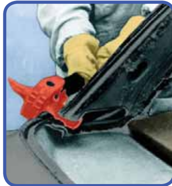
2. Cut off the roof pillars.
